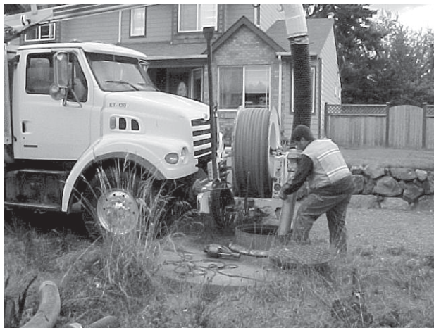
Crews with vector trucks cleaned out catch basins and storm lines to remove debris and roots from storm drainage pipes, ensuring that existing drainage systems work to their peak potential.
