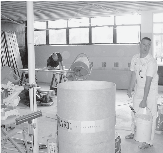
Improvements to Spartan Gym are expected to be complete in April.
