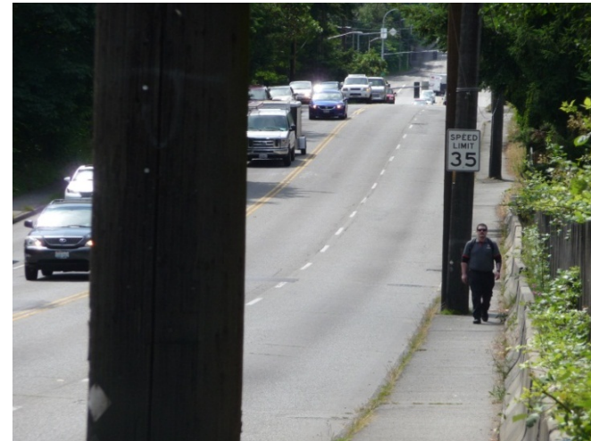
Narrow and non-ADA compliant sidewalk facilities along NE 145th Street near 10th Avenue NE
