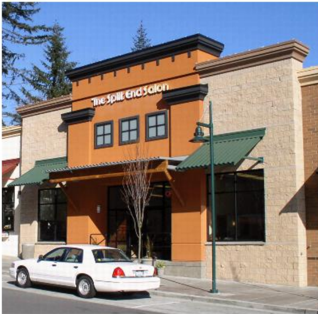
Concrete near the ground level and a variety of other surface materials on the facade.
