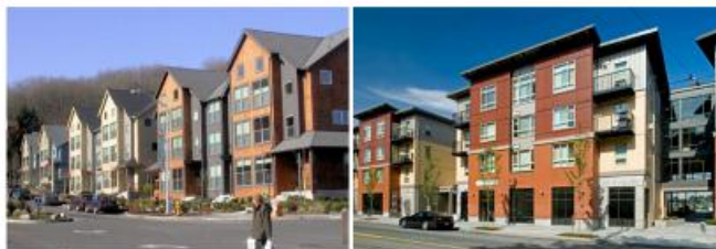
Multifamily building articulation
