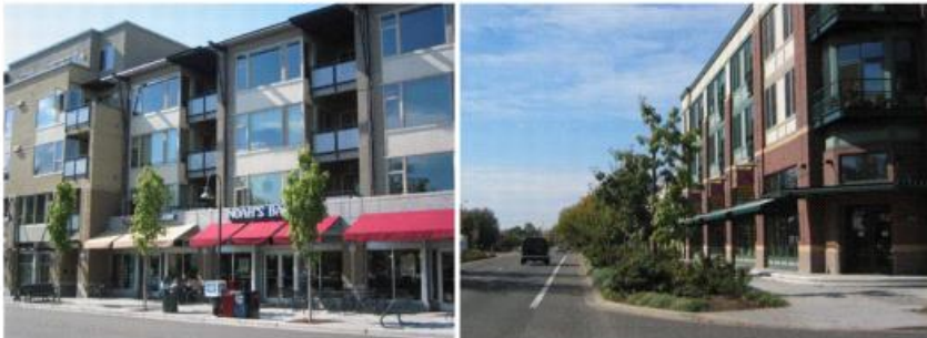
Storefront and boulevard buildings
