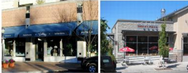
The left image uses smooth gray blocks on the vertical columns and beige split-faced blocks above the awnings. The storefront in the right image uses gray split face and some lighter, square, smooth-faced blocks below the storefront windows.
