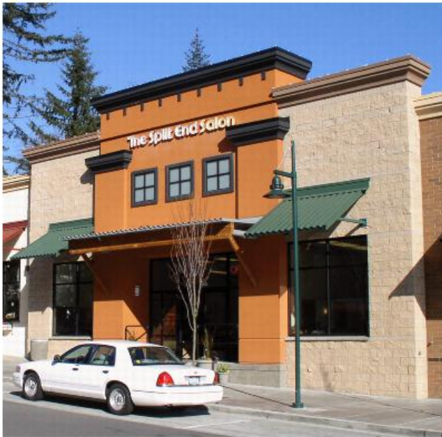
Concrete near the ground level and a variety of other surface materials on the facade.
