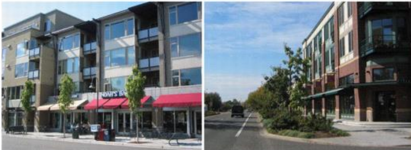
Storefront and boulevard buildings
