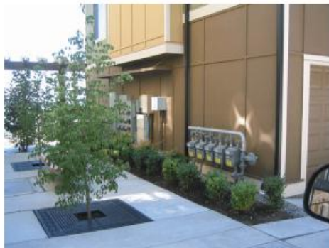
Utilities consolidated and separated by landscaping elements.
