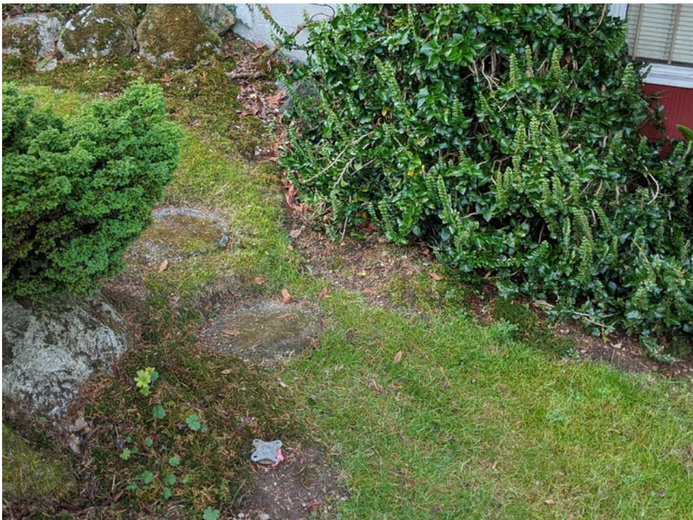
Looking west at the fuel port for a heating oil UST at the northeast corner of the house at address 2142 N 147th St.
