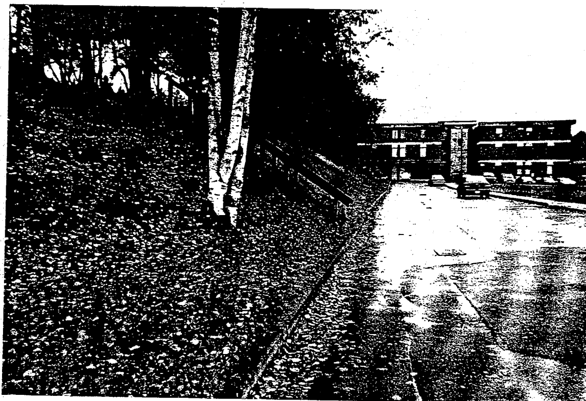
Photograph 2. Steep slope along the eastern side of the ridge at the western side of the site. The view is northeast toward Building 200 from the southern end of the ridge. The slope is up to 40 percent and ranges up to 20 feet, north of Building 200 in the mid-ground. The slope was cut during site development.
