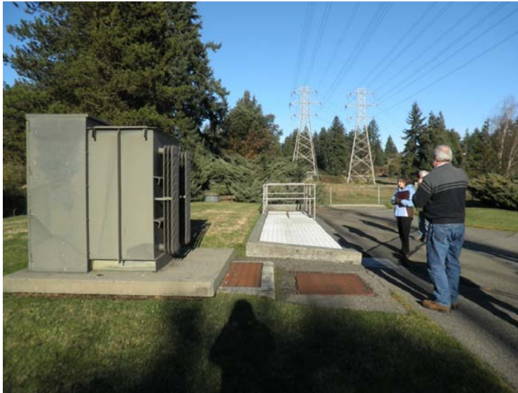
Figure 7 – North City Pump Station Exterior
