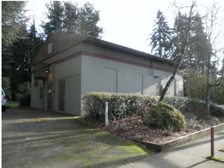
Figure 9 – Foy Pump Station Exterior
