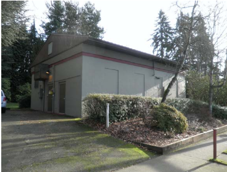
Figure 9 – Foy Pump Station Exterior
