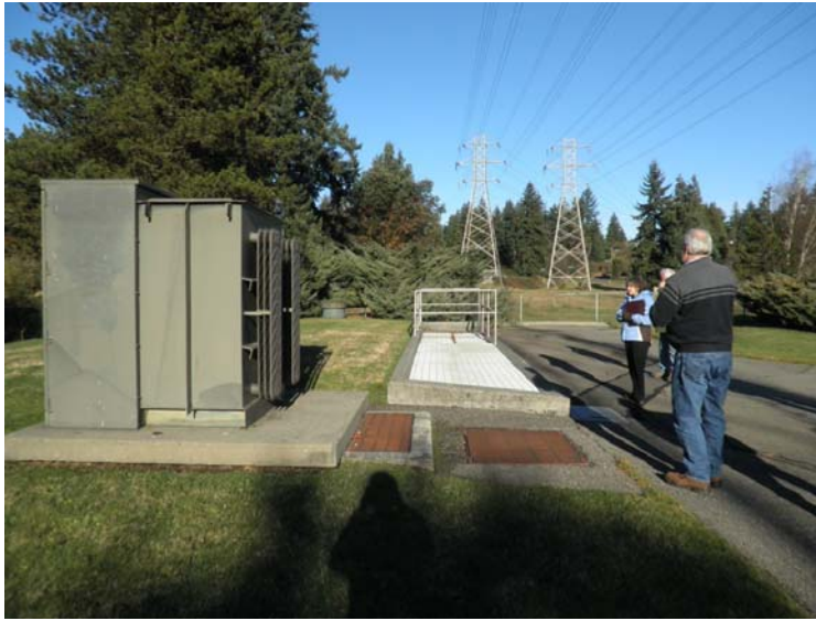
Figure 7 – North City Pump Station Exterior
