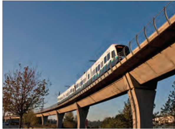
Elevated Light Rail Train with Overhead Catenary Wires
