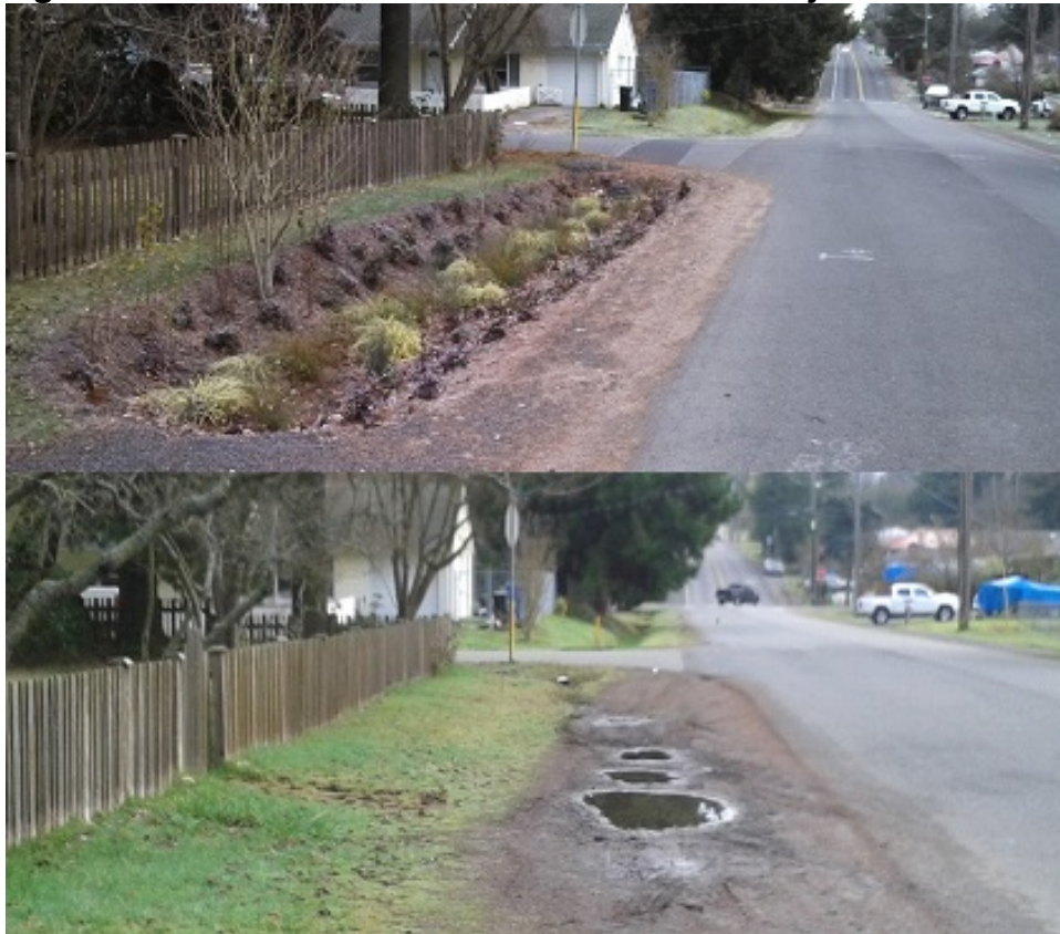
Figure 1. Bioretention Cell Before and After Project Photo.
