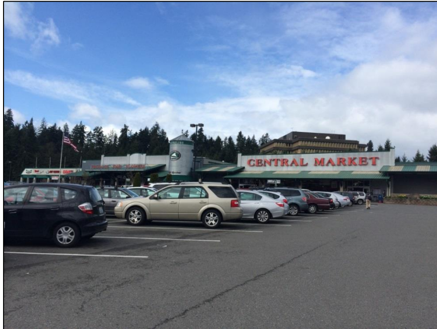
Figure 2-3. Current Site Photos: Commercial Areas Facing West (upper) and South (lower)
