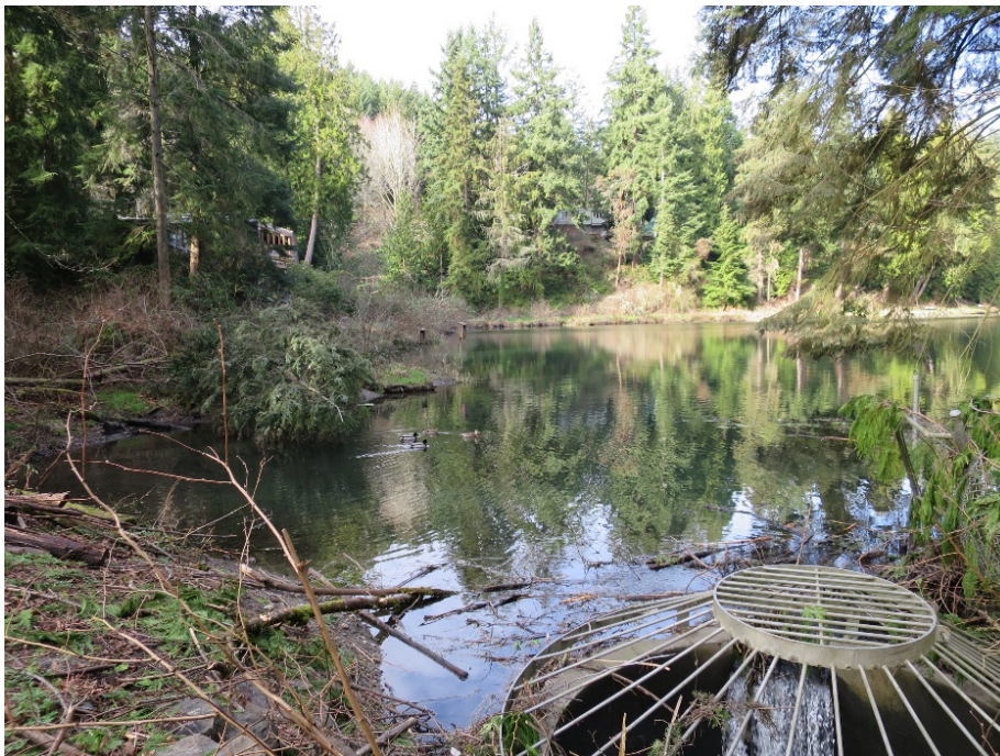
Figure 1. Existing Lake Outlet Structure as Viewed from the Dam.
