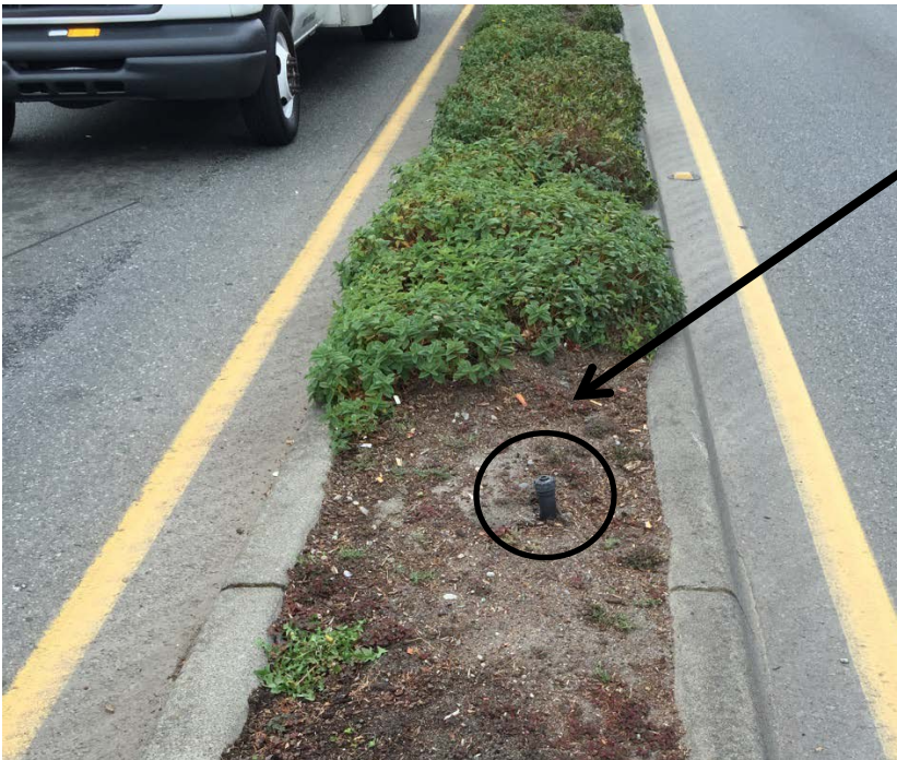
Photo 4 Example of pop-up sprinkler for corridor landscape watering.
