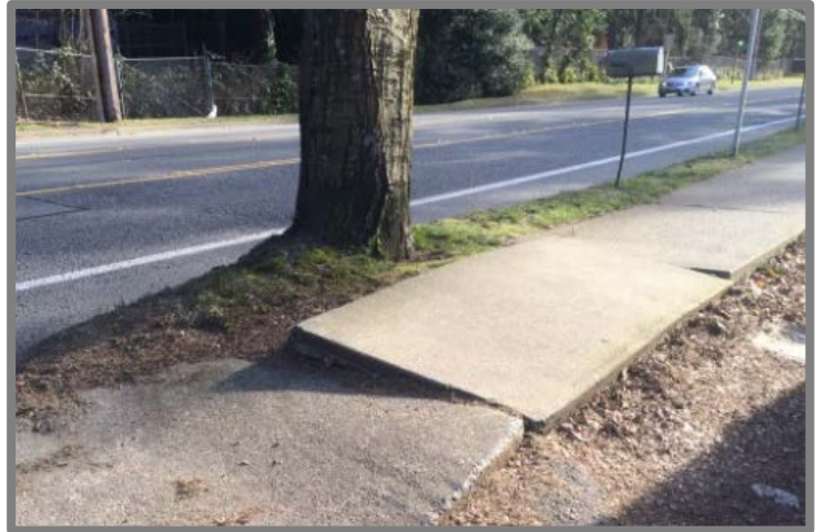
Sidewalk damaged by tree roots
