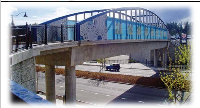
Interurban Trail Bridges , Vicki Scuri, artist concrete, steel, glass, light and greening 155th Ave N at Aurora Ave N and Aurora Ave N at 160th City of Shoreline 1% for Art Program 2007
