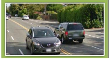
**Proposed Roadway:** Two way left turn lane is unoccupied most of the time. More separation between the main streams of traffic. Drivers typically slow as they enter the turn lane, making it easier to adapt to opposing traffic, and less catastrophic in the event of collision.
