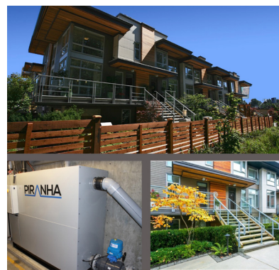
Figure 5 — Building Scale Sewer Heat Recovery
