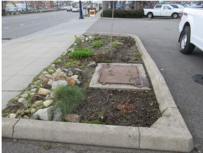
Figure 4-16. Oil/water separator
