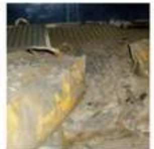
Figure 2. Perlite filter media needs replacement.
