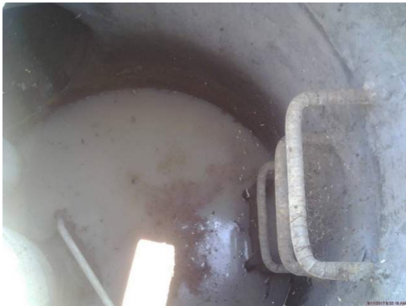
Figure 5-1. Illicit discharge of wet concrete in manhole
