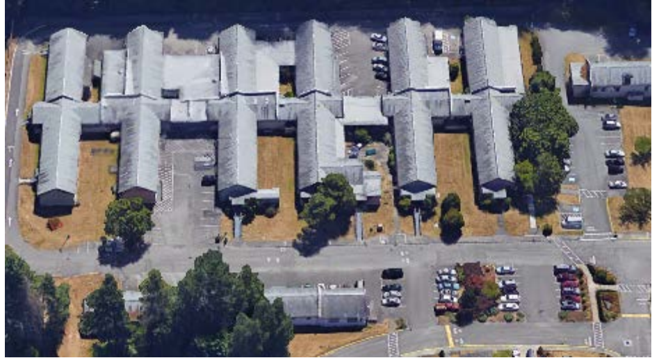
Figure 9: Existing ATP Building
