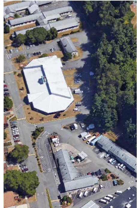
Figure 12: Existing Kitchen Building (middle) and Steam Plant (bottom center)
