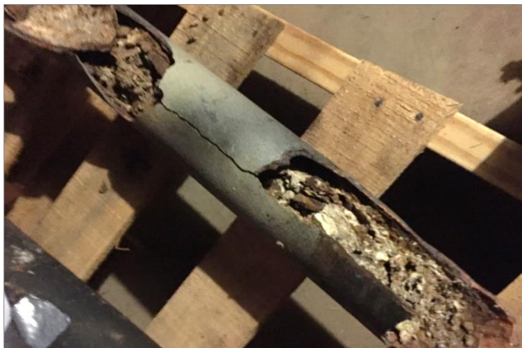
Figure 1. Waste Pipe from Skilled Nursing Building
