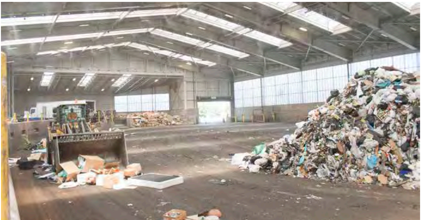
Bow Lake Recycling and Transfer Station
