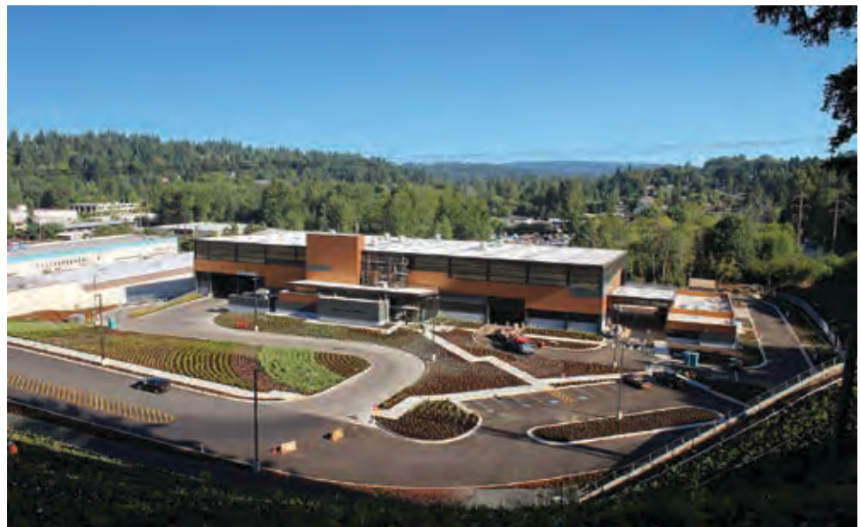
The new Factoria Recycling and Transfer Station opened in the fall of 2017
