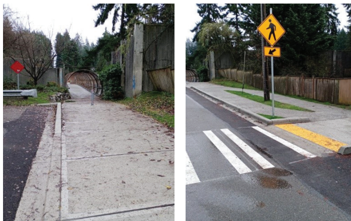
Left: The shared-use sidewalk to the pedestrian bridge over I-5. Right: The new crosswalk and curb ramp.
