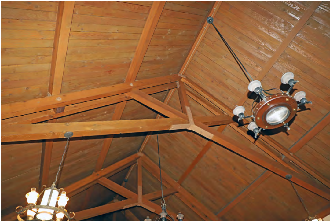
Figure 51. Truss and branched fixture detail.
