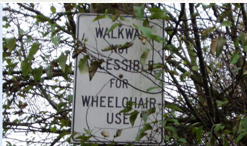
Substandard sidewalks, high accident rates, and high traffic volumes create safety challenges for all users of 145 th Street
