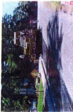
A fog seal is applied after the BST has cured
