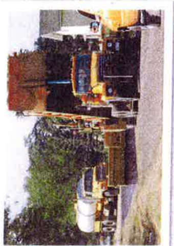
Asphalt and chips are applied to the existing pavement
