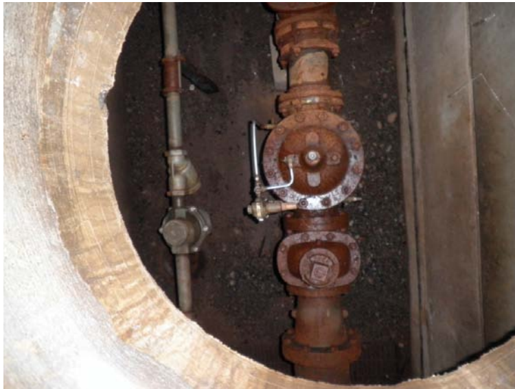
Figure 8 – Pressure Reducing Valve, 9th Ave NW & Innes Arden Way
