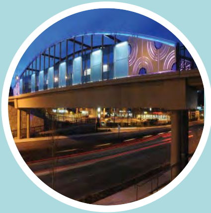
Aurora Avenue N Bridge
