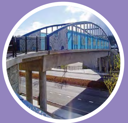
Auroa Pedestrian Bridge
