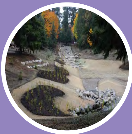
Boeing Creek Stormwater Improvements
