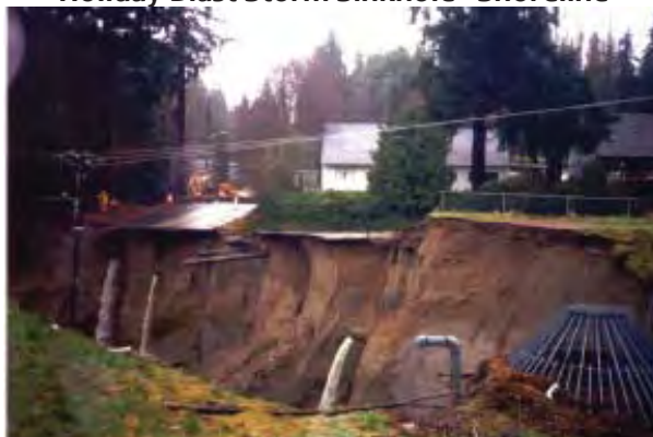
Figure NEA-2 Holiday Blast Storm Sinkhole - Shoreline
