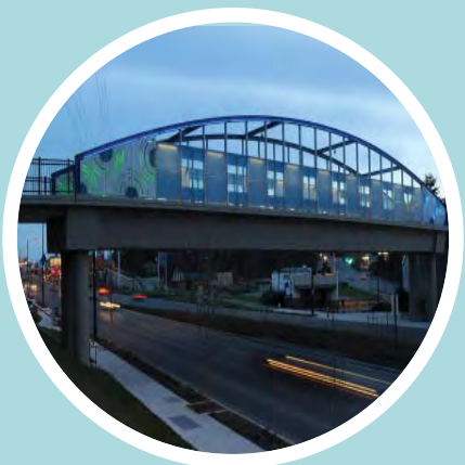
Aurora Avenue N Bridge
