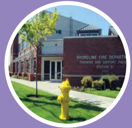
Shoreline Fire Station
