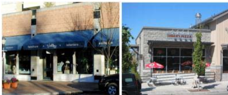
The left image uses smooth gray blocks on the vertical columns and beige split-faced blocks above the awnings. The storefront in the right image uses gray split face and some lighter, square, smooth-faced blocks below the storefront windows.
