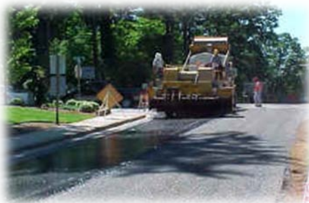
A fog seal is applied after the BST has cured
