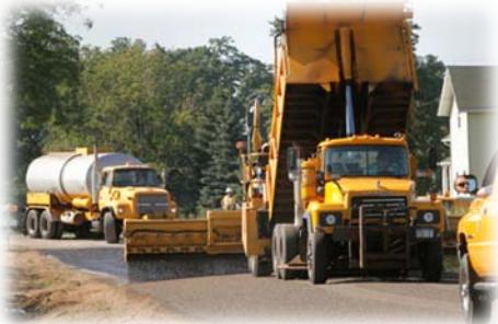
Asphalt and chips are applied to the existing pavement
