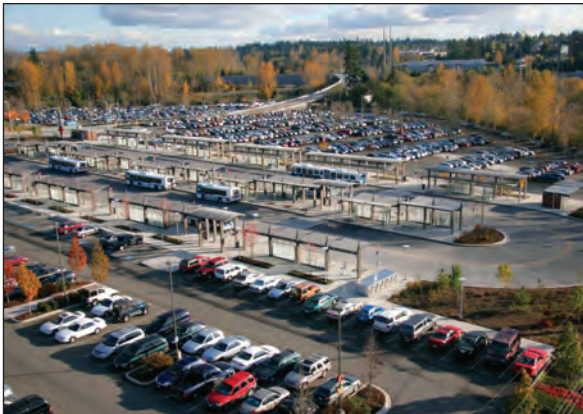
Lynnwood Transit Center
