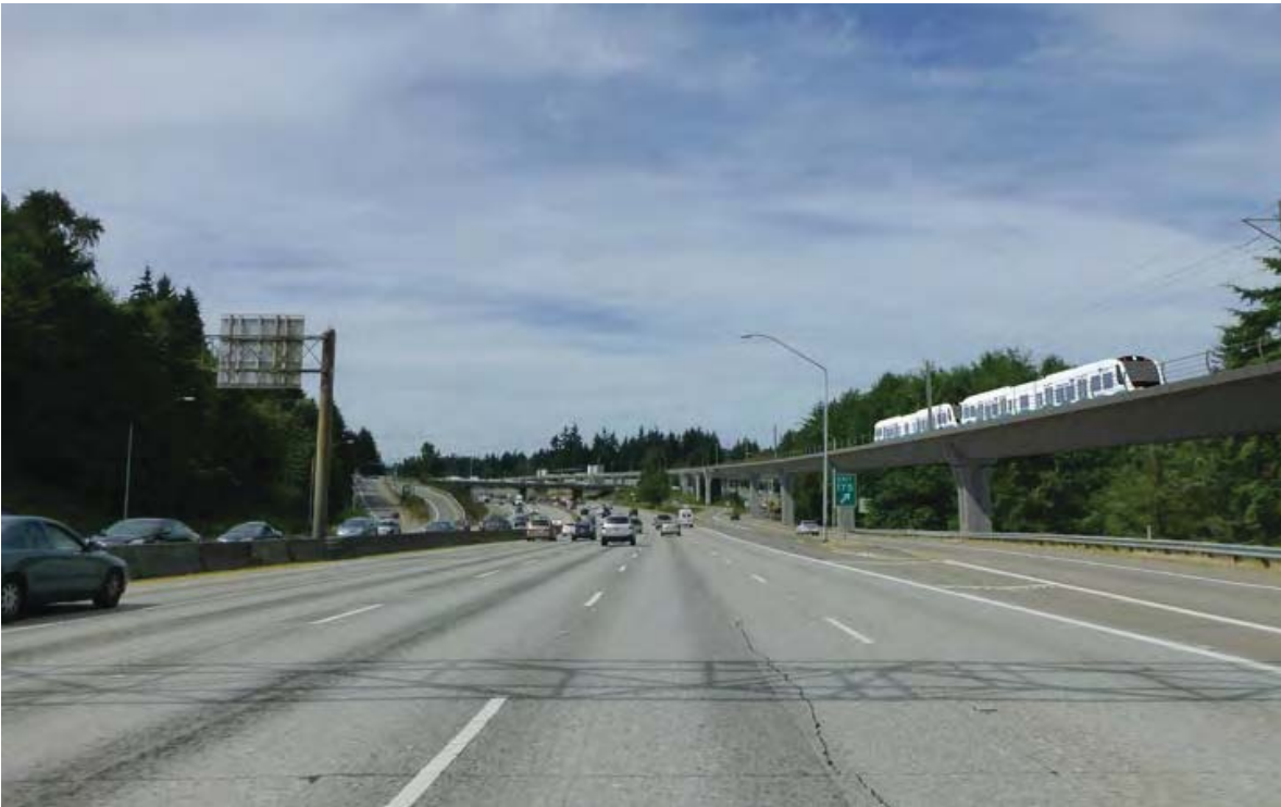
Figure G-34. Viewpoint 10 I-5 Northbound at NE 143rd Street View to the north Simulation: Alternatives A1 and A10
