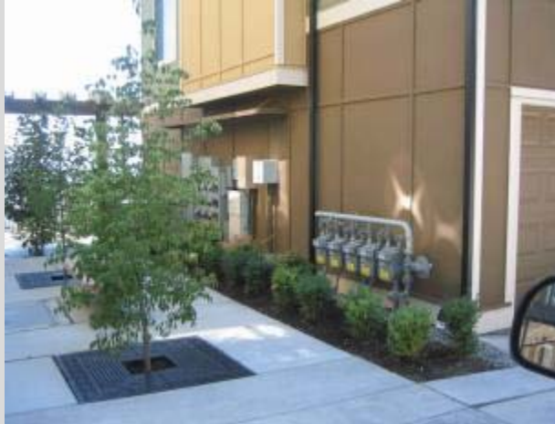
Utilities Consolidated and Separated by Landscaping Elements
