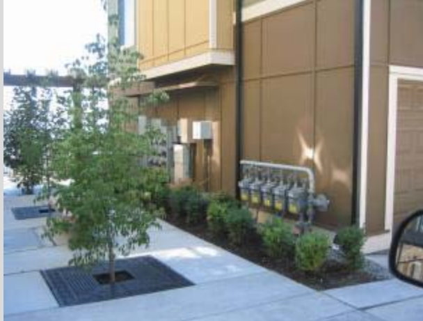
Utilities Consolidated and Separated by Landscaping Elements
