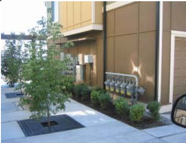
Utilities Consolidated and Separated by Landscaping Elements
