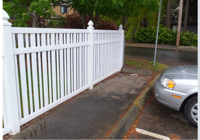
Abrupt sidewalk end at the south edge of Westminster Manor property.
