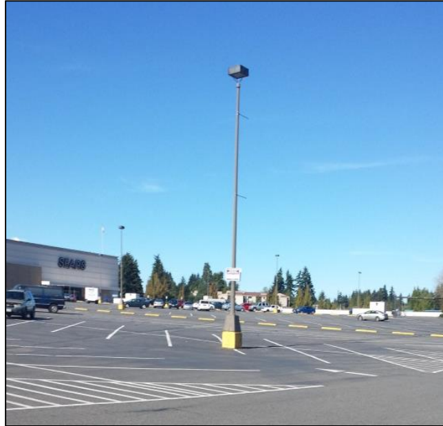
Figure 3-6. Light in surface parking lot
