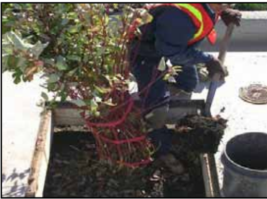
3. Removal of debris, trash and mulch
