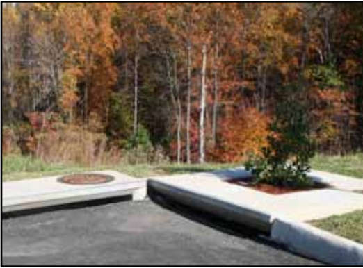
1. Inspection of Bioretention Box and surrounding area
