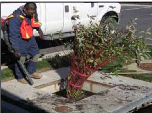
5. Clean area around Bioretention Box
