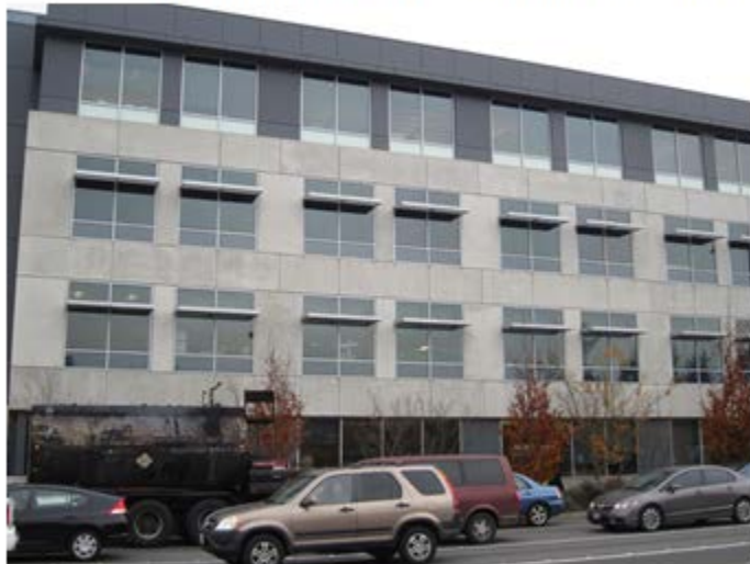
Approximately 35% Windows Coverage
