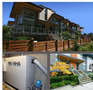
Figure 5 — Building Scale Sewer Heat Recovery
