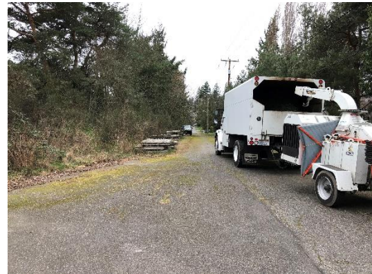
Looking west from monopole towards gate
