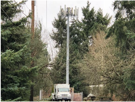
View of subject looking W from access gate
