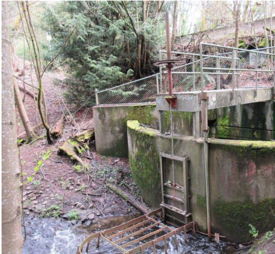
Figure 4-11. Gate valve
