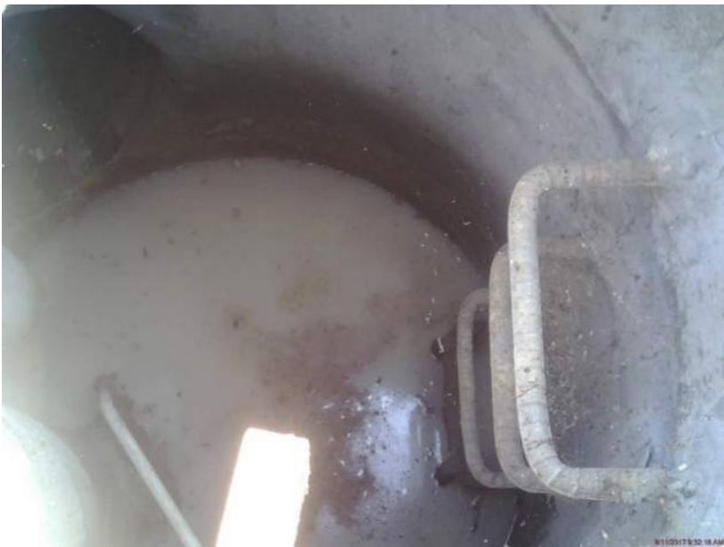
Figure 5-1. Illicit discharge of wet concrete in manhole
