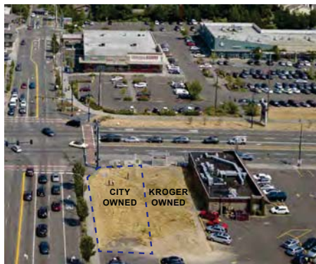
AERIAL VIEW OF SITE
