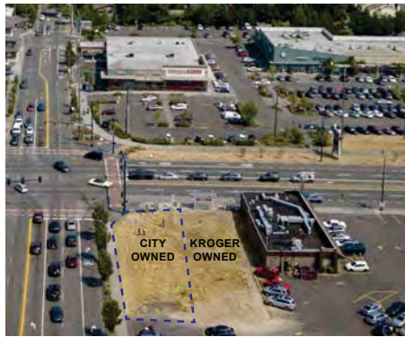
AERIAL VIEW OF SITE
