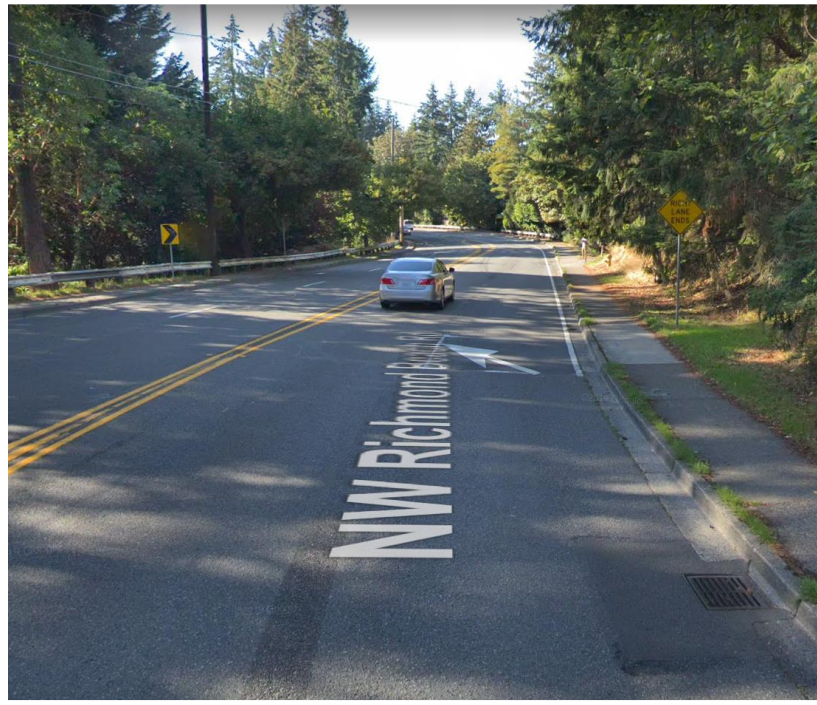
Figure 8 – Westbound merge between Dayton Ave N and 3 rd Ave NW
