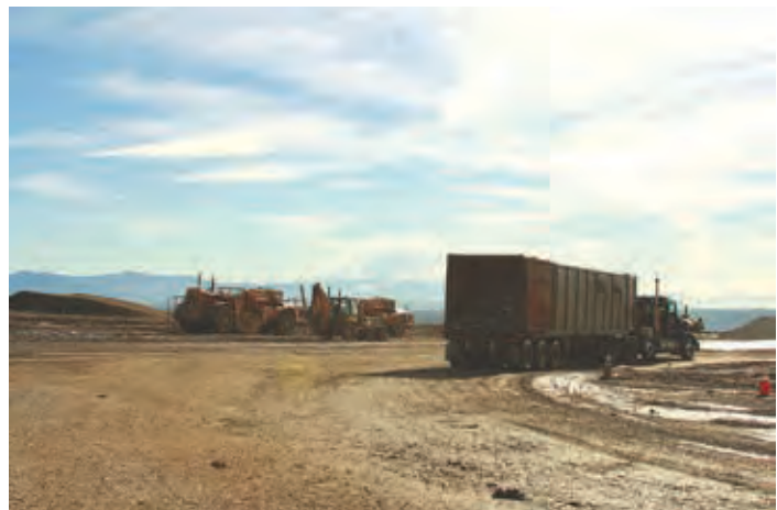
The CERP Fund provides resources for replacement and major maintenance of equipment
