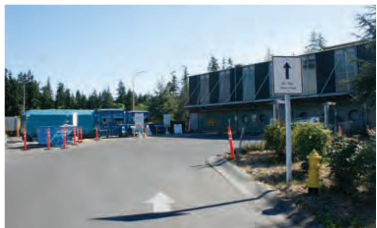
The Vashon Recycling and Transfer Station
