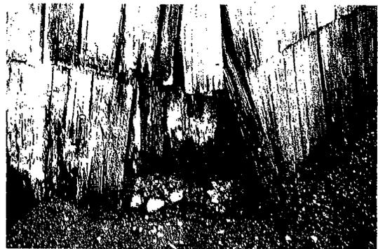
foundation to be structurally sound for reuse. In the event an agreement is not achieved then the existing foundation would need to be removed and replaced with a new structurally designed system. In essence the tower would be dismantled, all dry rotted wood replaced, the foundation removed and replaced, and finally the tower reconstructed over the new foundation.
