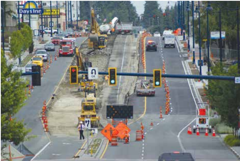
Demolishing the center lanes before beginning median construction
