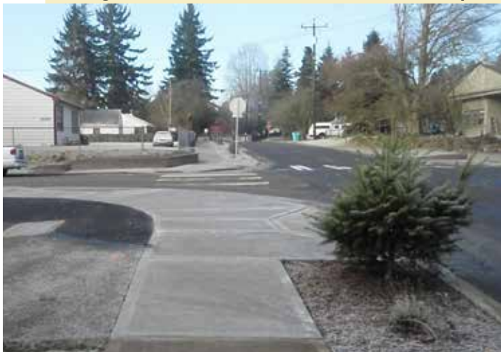
Below and right: New sidewalks near Briarcrest Elementary
