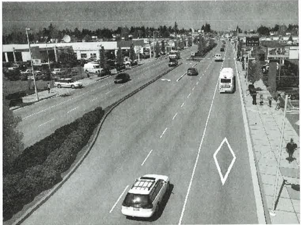
This computerized view of Aurora from 170th looking north shows business access/transit lanes, a combined sidewalk/landscape strip and landscaped medians. The medians have left turn and u-turn pockets every 800 to 1,000 feet and offer a safety zone for pedestrians to cross.
