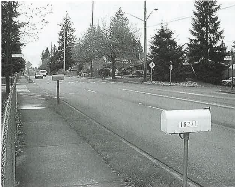
The new signal will make it safer for traffic entering 15th Ave. NE from N. 165th St.
