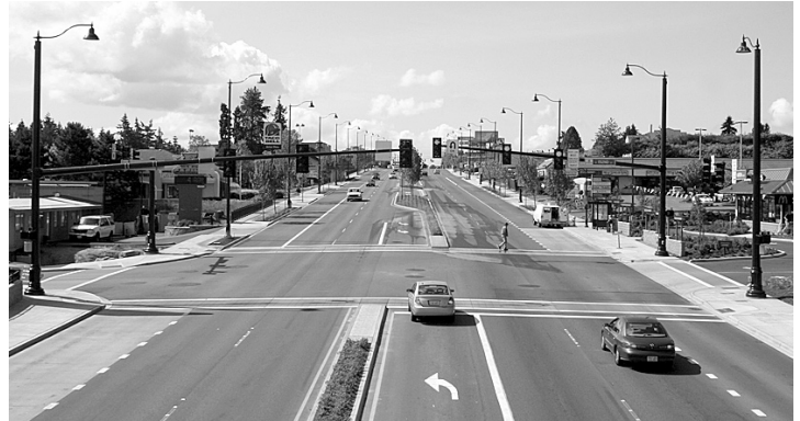
The photo above shows the intersection at N 152nd Street and Aurora looking south. The City of Shoreline celebrated the completion of its first mile of Aurora from N 145th to N 165th Streets earlier this year. Planning and design is already underway to improve the next two miles from N 165th to N 205th Streets.
