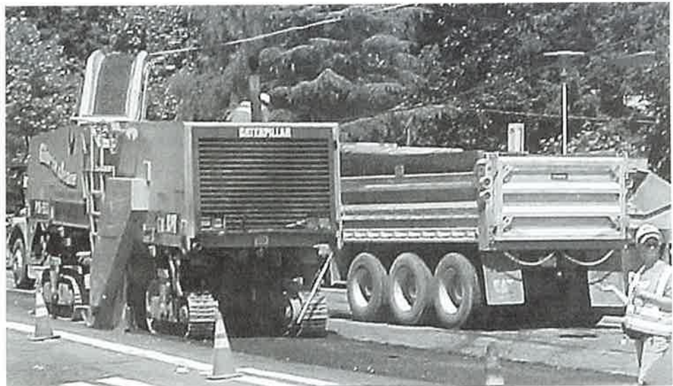
The grinding process on 175th took crews two days to complete.
